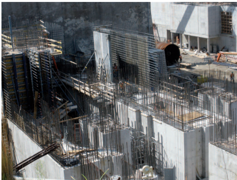
Construction work at New York's new UV treatment facility. Courtesy NYCDEP.
