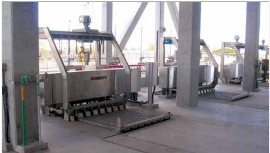
The TrojanUV4000Plus™ has been optimized for disinfection of low quality wastewater using high intensity lamps, and vortex mixers (left) to increase flow turbulence around the lamps. Trojan's UV technology allowed the City of Honolulu, Hawaii to disinfect primary effluent at their Sand Island treatment facility (right), and thereby save hundreds of millions of dollars that would have been required to build secondary treatment facilities.
