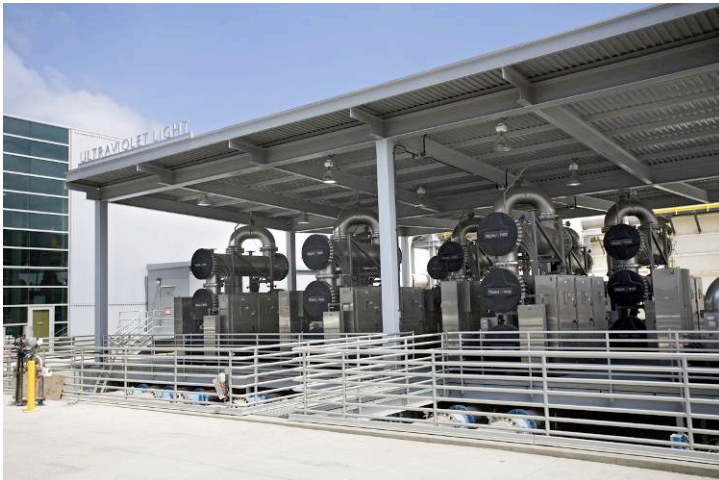
The TrojanUVPhox™: a key element of the Orange County Ground Water Replenishment system in California, USA.
