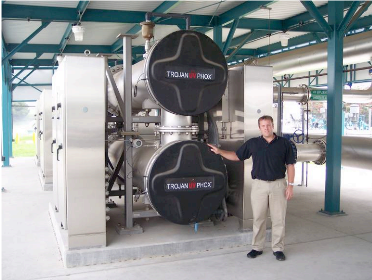
The two-chamber TrojanUVPhox™ treatment train at West Basin, California is similar to the configuration at Bundamba1A and 1B.
